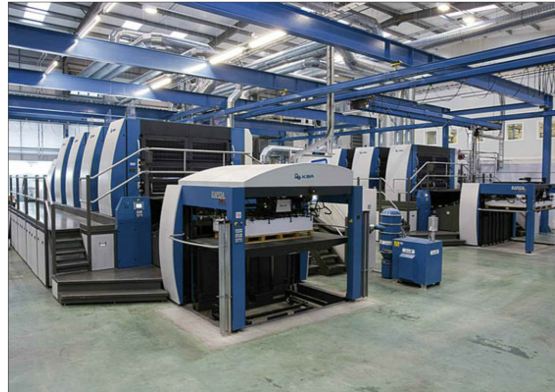
Two Rapida 205 press lines are in operation at Capital Print & Display's new production plant in London In der neu erbauten Fabrik von Capital Print & Display in London produzieren zwei KBA Rapida 205.
